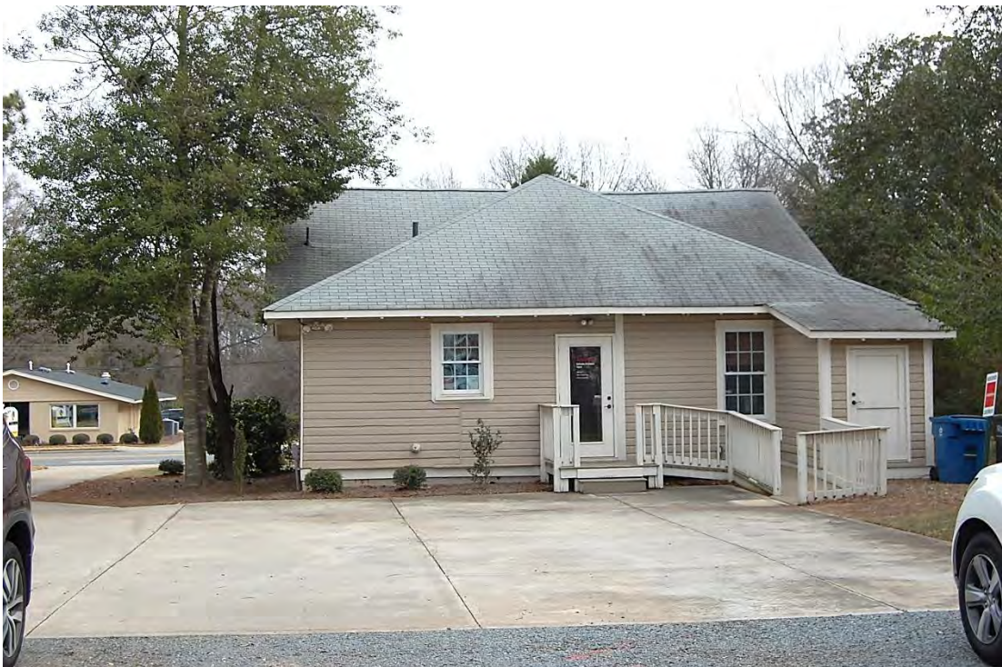
James and Martha Russell House No. 1, Rear (South) Elevation Looking Northeast.
