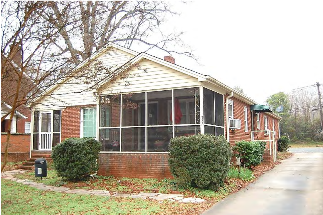
Duplex, 322-324 West John Street, Looking North.
