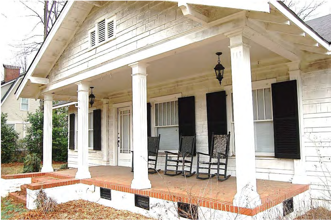
Henry and Hazeline Massey House, Front Porch, Looking North.
