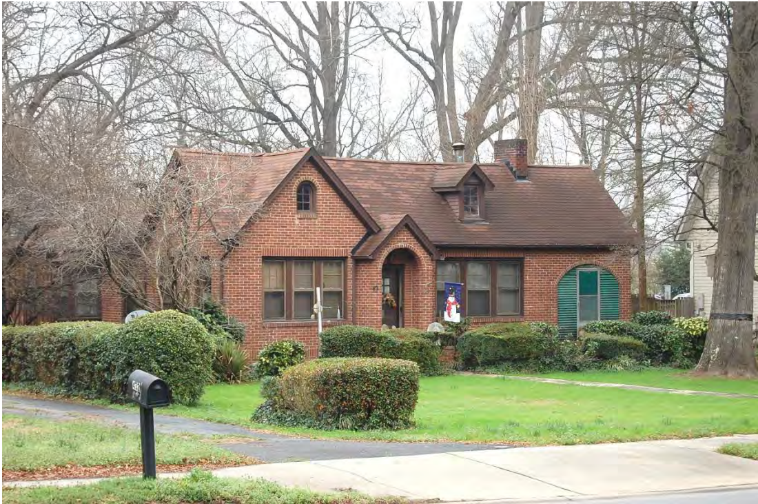
John and Roselie Stewart House, Overall View, Looking North.
