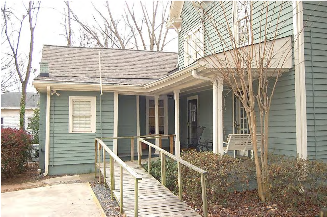
Grier-Furr House, Rear (East) Elevation, Looking South.
