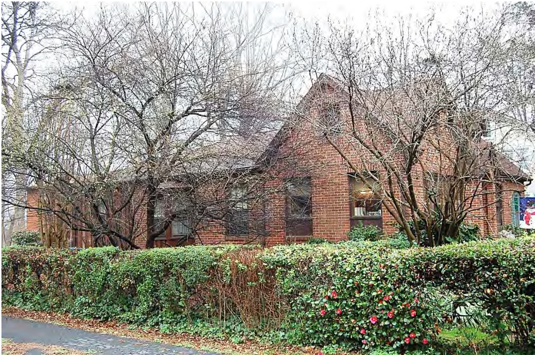
John and Roselie Stewart House, Side (West) Elevation, Looking Southeast.
