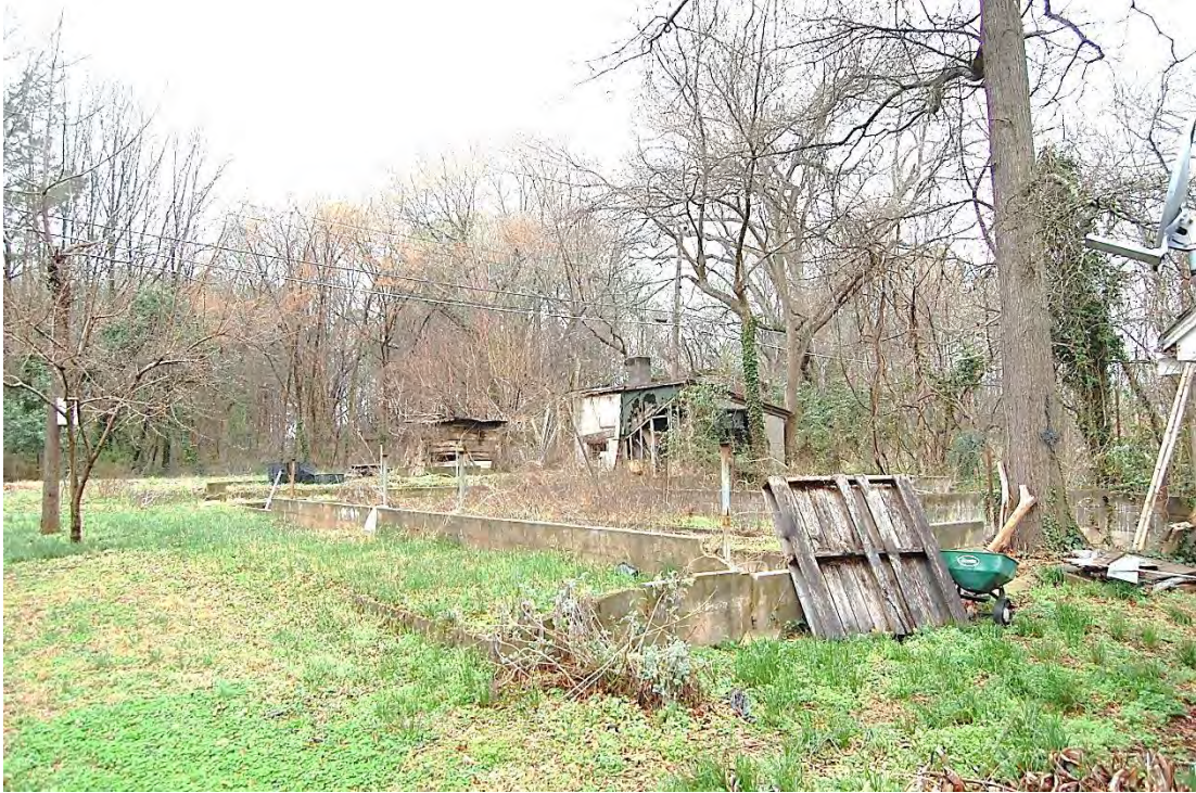
McLaughlin-Bost House, Ruinous Outbuildings, Looking Southwest.
