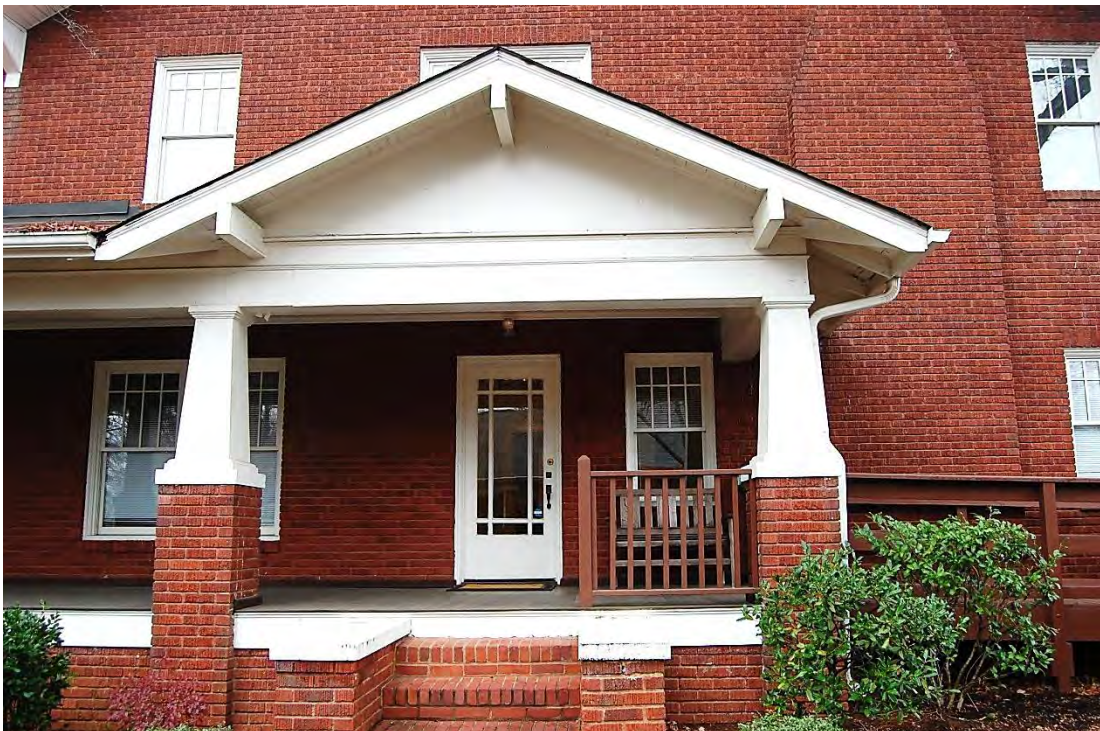
Renfrow-Lemmond House, Side (East) Elevation Showing Secondary Entrance, Looking West.
