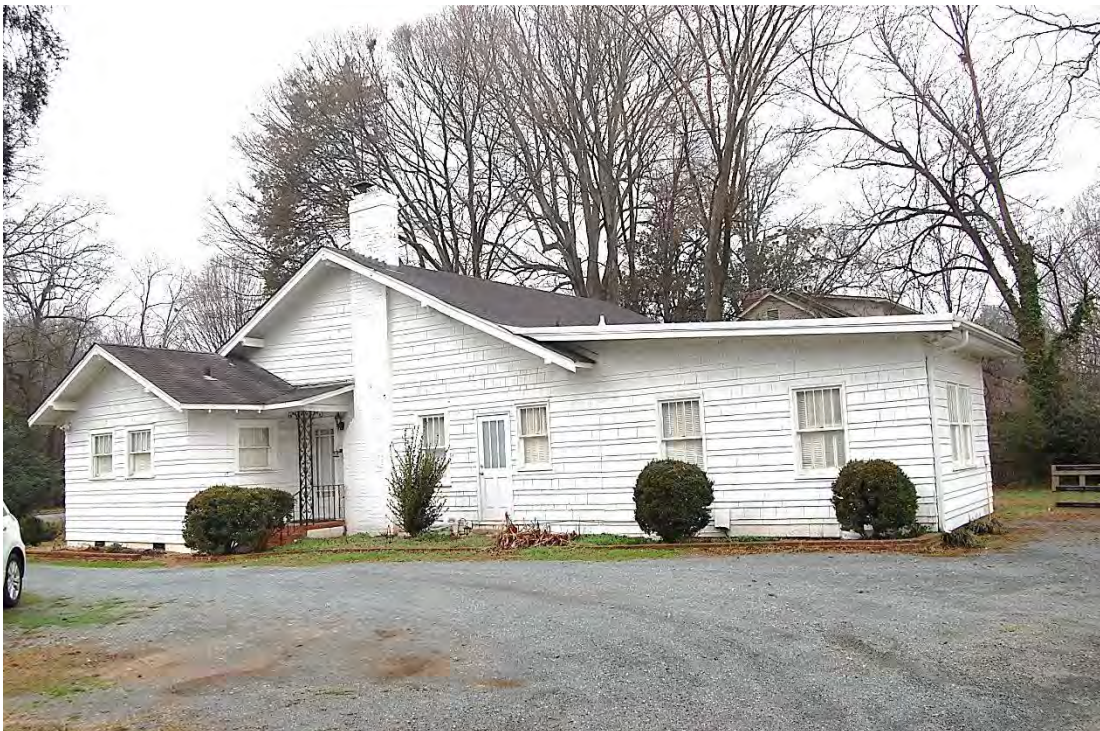
Henry and Hazeline Massey House, Side (East) Elevation and Rear Addition, Looking West.
