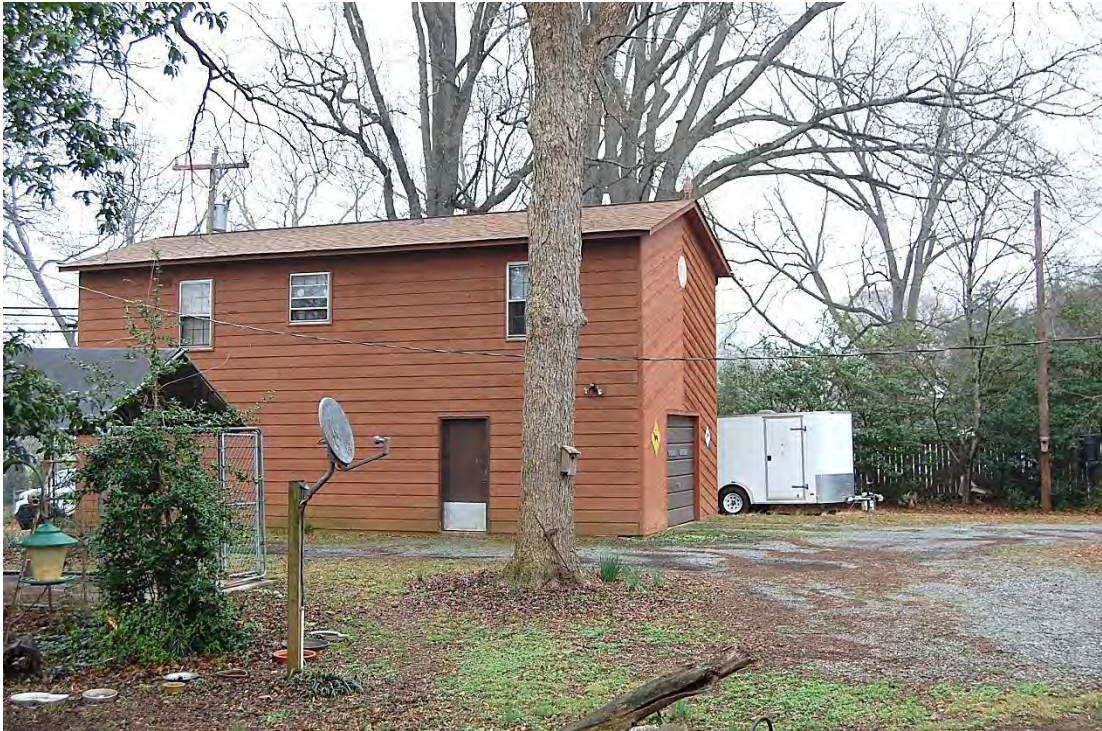
John and Roselie Stewart House, Modern Garage/Guest House, Looking East.
