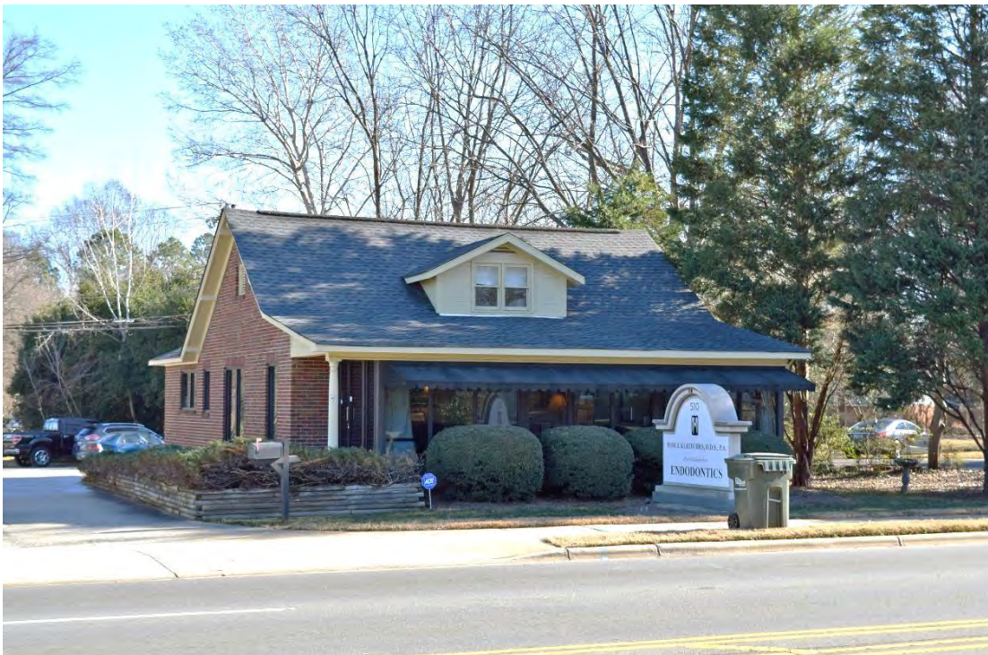
Jesse and Ethel Hartis House, Façade and North Elevation, Looking East.
