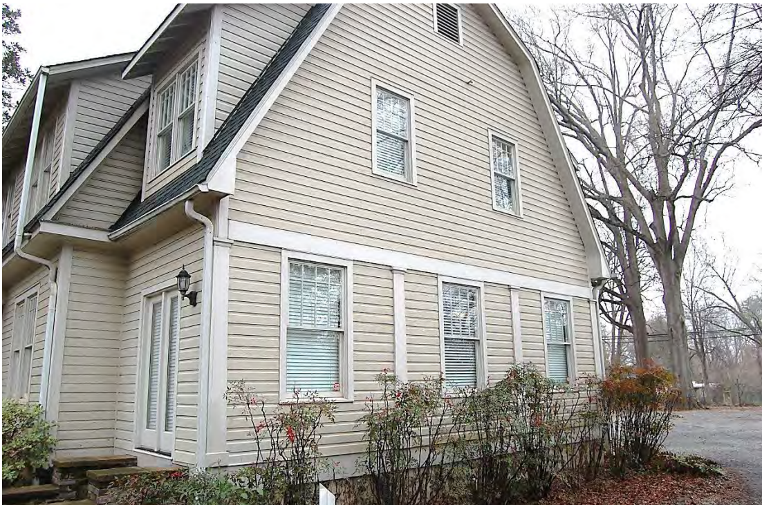
Kidd-Tennant-Roberts House, Enclosed Side Porch, Looking Northwest.
