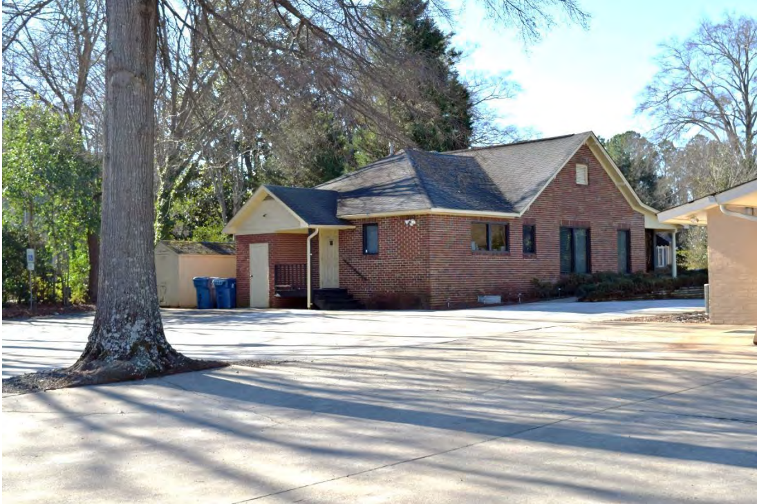
Jesse and Ethel Hartis House, Rear (North) and Side (West) Elevations, Looking South.
