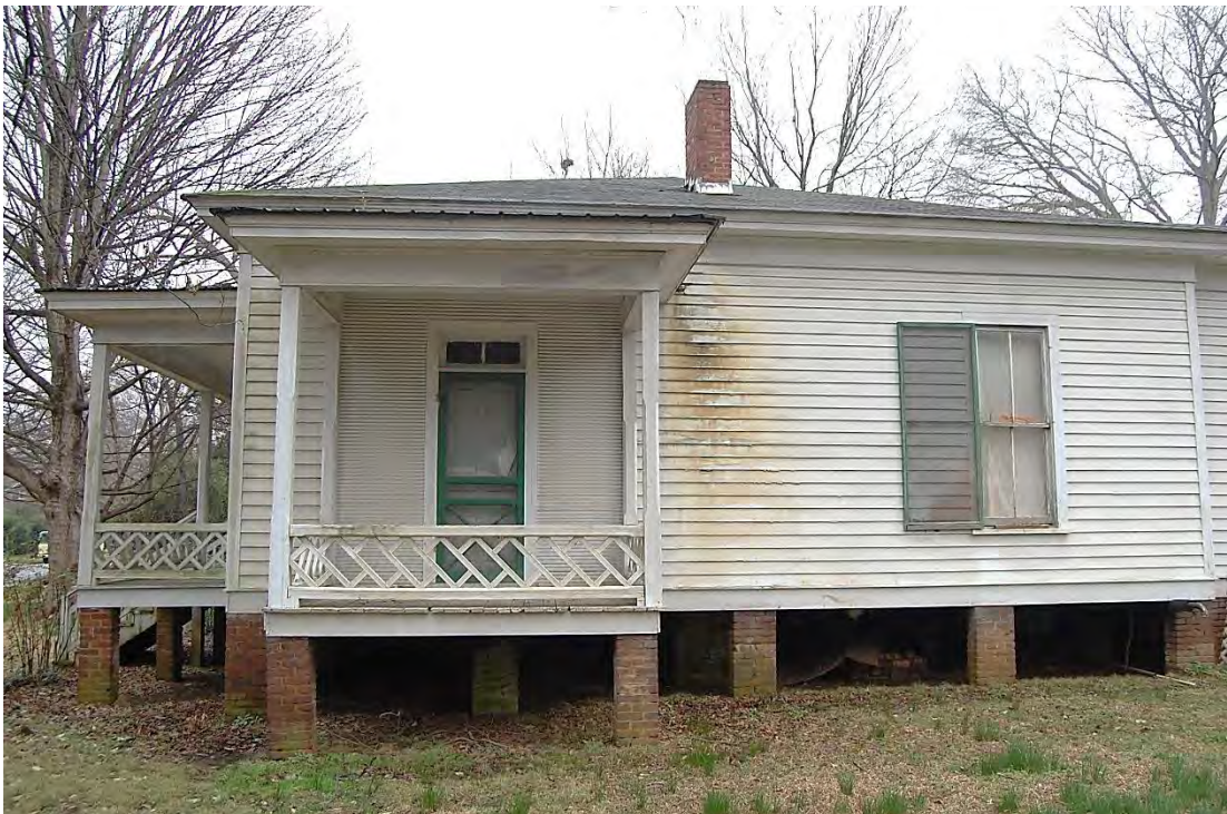
McLaughlin-Bost House, Side (West) Elevation, Porch, Looking East.
