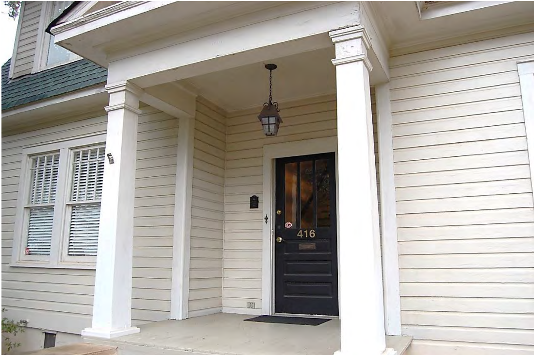
Kidd-Tennant-Roberts House, Front Entrance, Looking Northwest.
