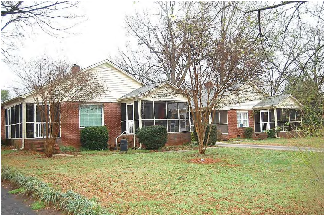
Duplex, Overall View, 322-324 West John Street (Left) and 316-318 West John Street (Right), Looking Northeast.
