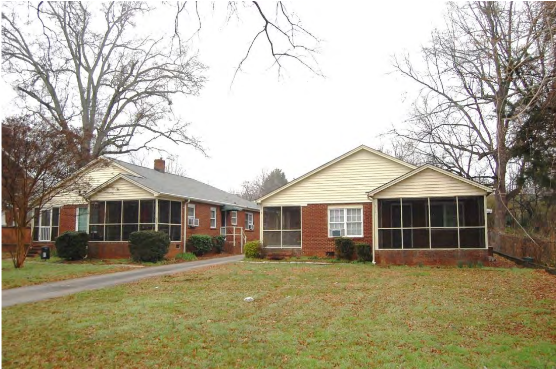
Duplex, Overall View, 316-318 West John Street (Right) and 322-324 West John Street (Left), Looking North.
