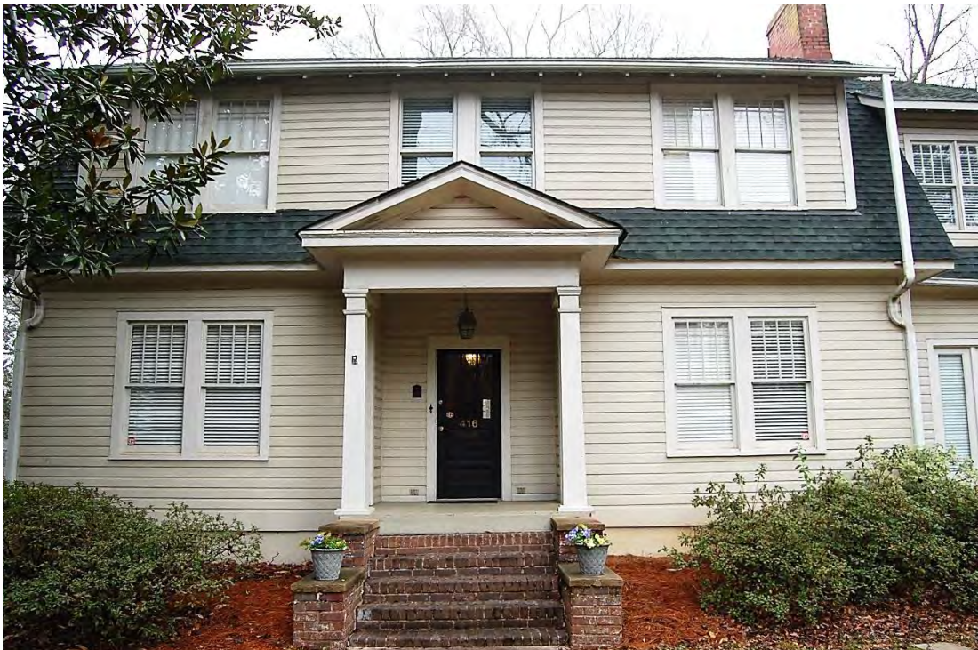
Kidd-Tennant-Roberts House, Façade, Looking North.
