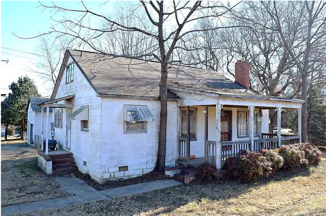
Haigler-Privette House, Façade, Looking East.
