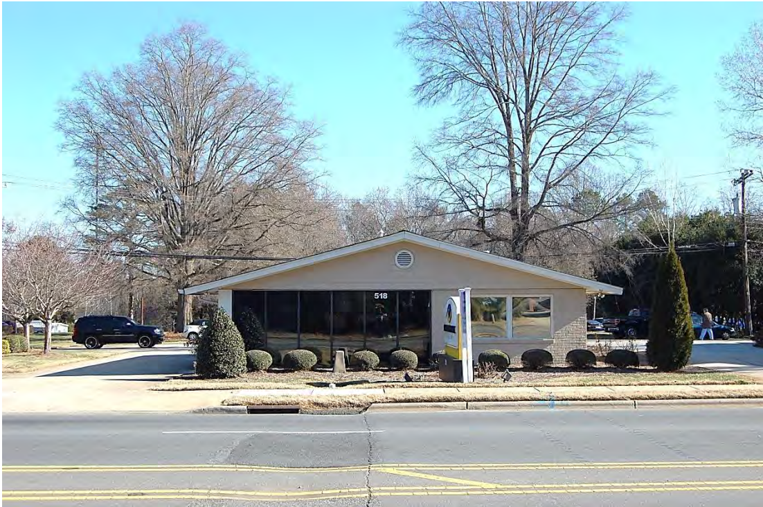
Medical Office Building, Façade, Looking Northeast.
