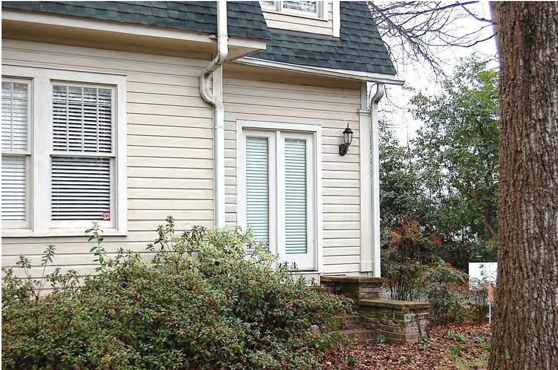
Kidd-Tennant-Roberts House, Façade and Enclosed Side Porch, Looking Northeast.
