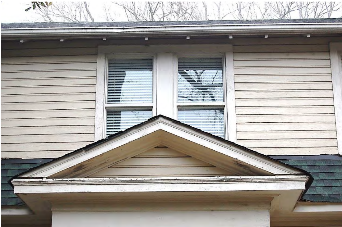
Kidd-Tennant-Roberts House, Façade, Replacement Windows Above Entrance Porch, Looking North.
