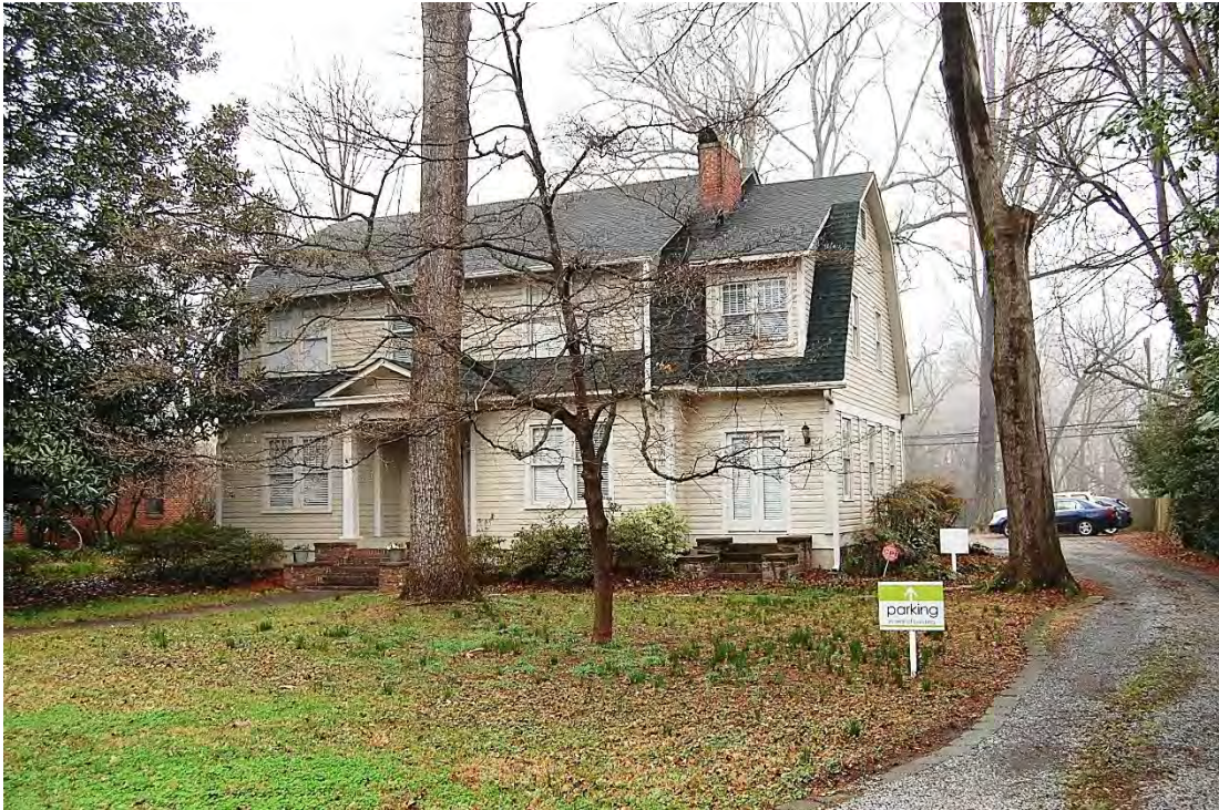
Kidd-Tennant-Roberts House, Overall View of House and Setting, Looking North.
