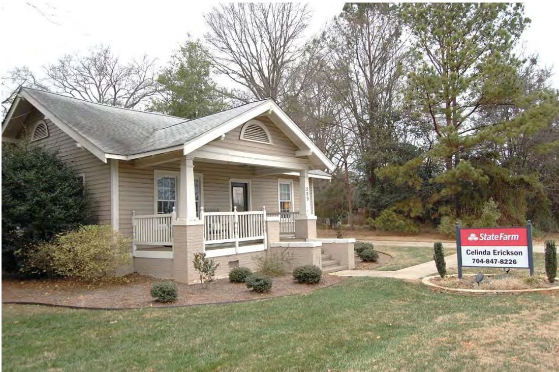
James and Martha Russell House No. 1, Façade and Side (East) Elevation, Looking Northwest.
