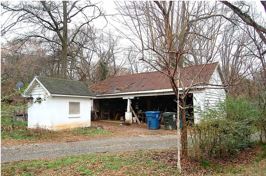
McLaughlin-Bost House, Equipment Storage Shed and Pump House, Looking Southwest.
