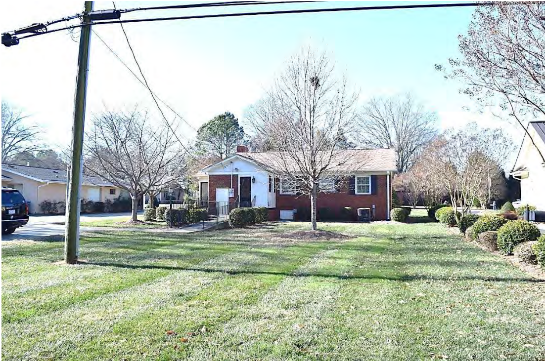
Dora Culledge House, Rear (East) Elevation, Looking West.
