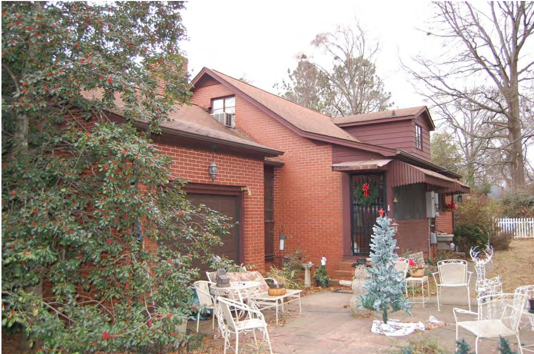
James and Martha Russell House No. 2, Rear (South) Elevation, Looking Southeast.
