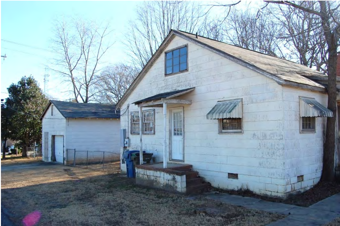
Haigler-Privette House, Side (West) Elevation, and Garage, Looking Southeast.
