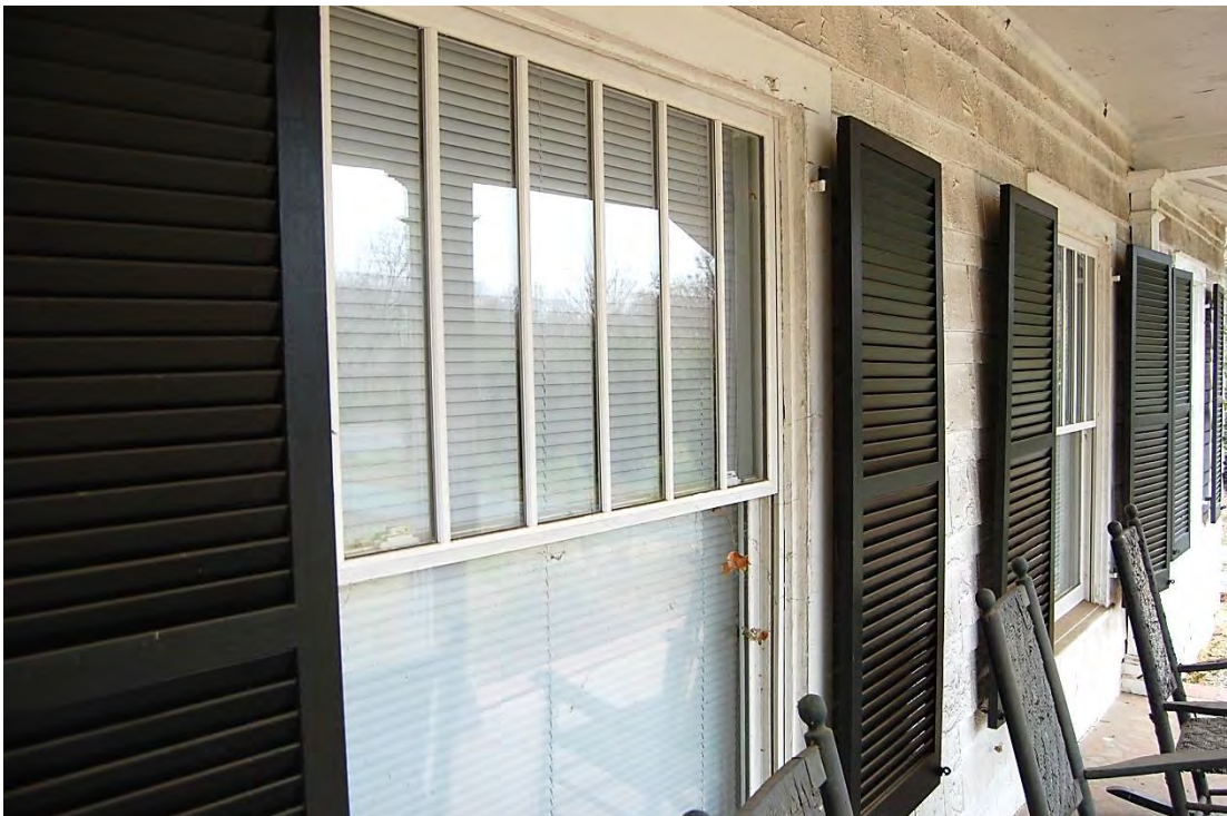
Henry and Hazeline Massey House, Façade, Replacement Window.
