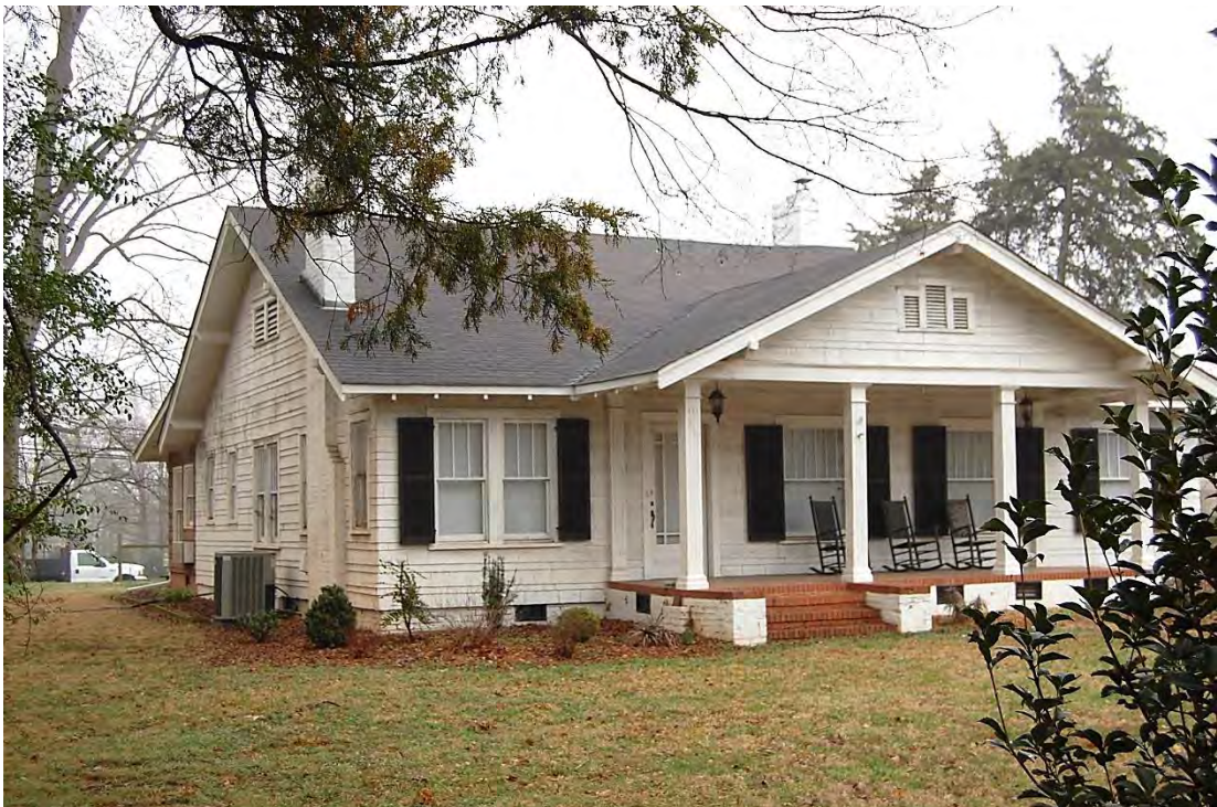
Henry and Hazeline Massey House, Façade and Side (West) Elevation, Looking North.
