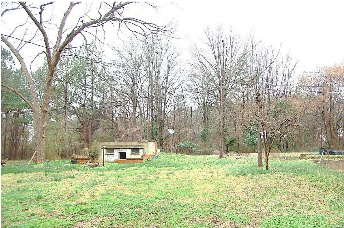
McLaughlin-Bost House, Ruinous Concrete Block Potato House, Looking South From House.
