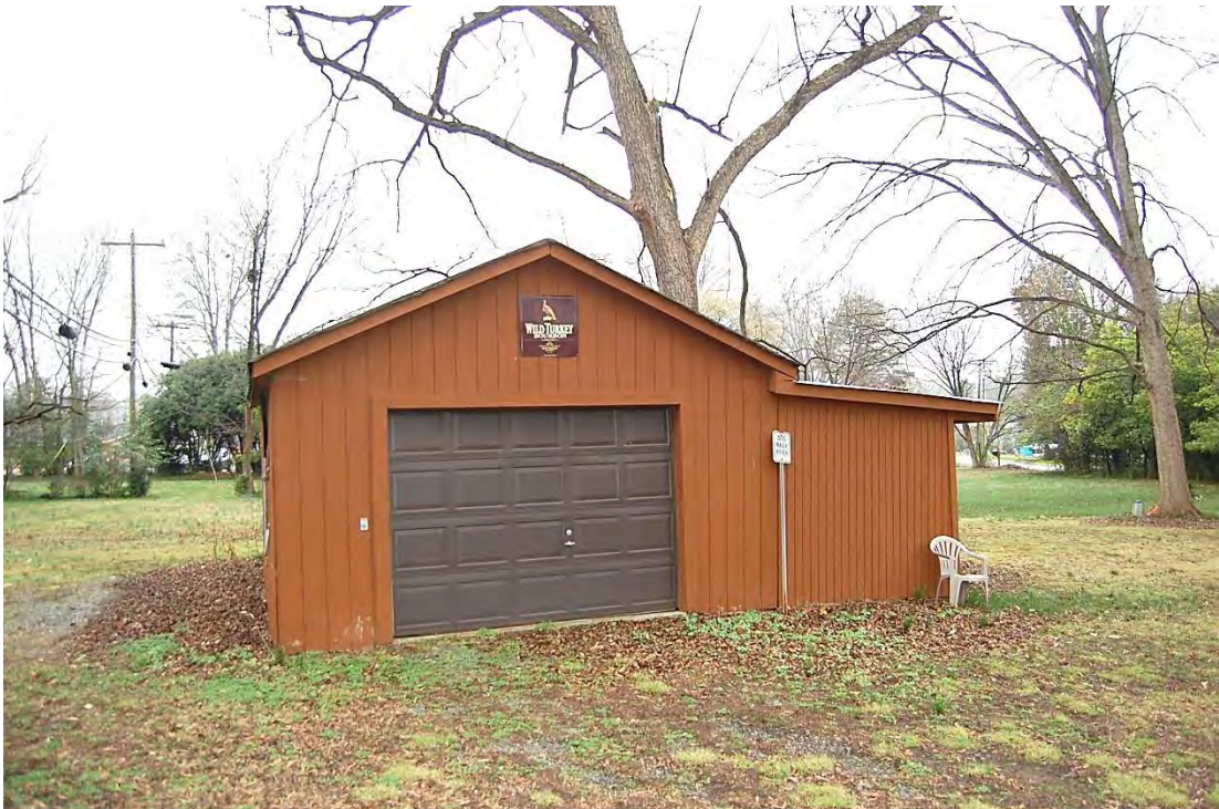
John and Roselie Stewart House, Modern Garage, Looking Northwest.
