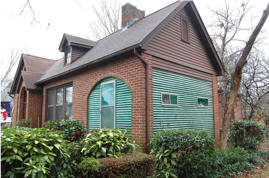
John and Roselie Stewart House, Façade and Side (East) Elevations, Looking North.
