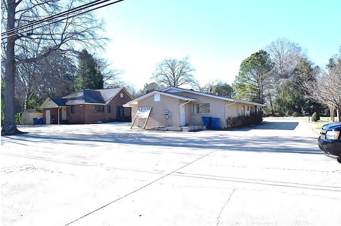
Medical Office Building, Rear (North) Elevation, Looking Southwest.
