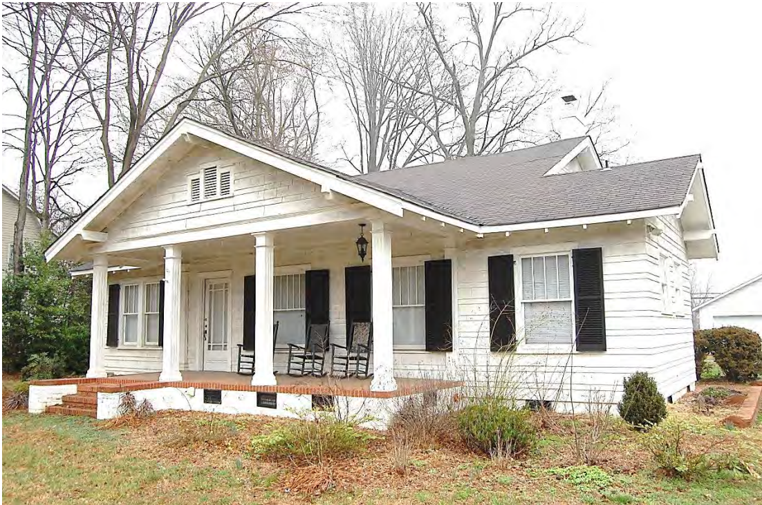
Henry and Hazeline Massey House, Façade, Looking North.
