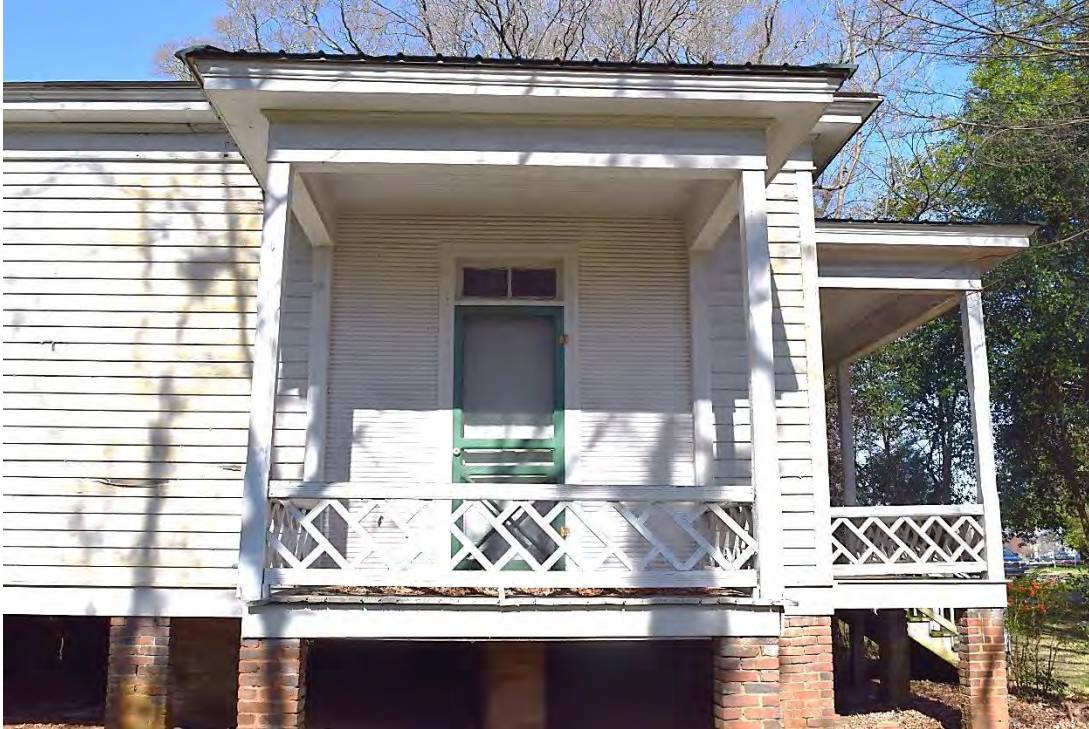
McLaughlin-Bost House, Side (East) Elevation, Porch, Looking West.
