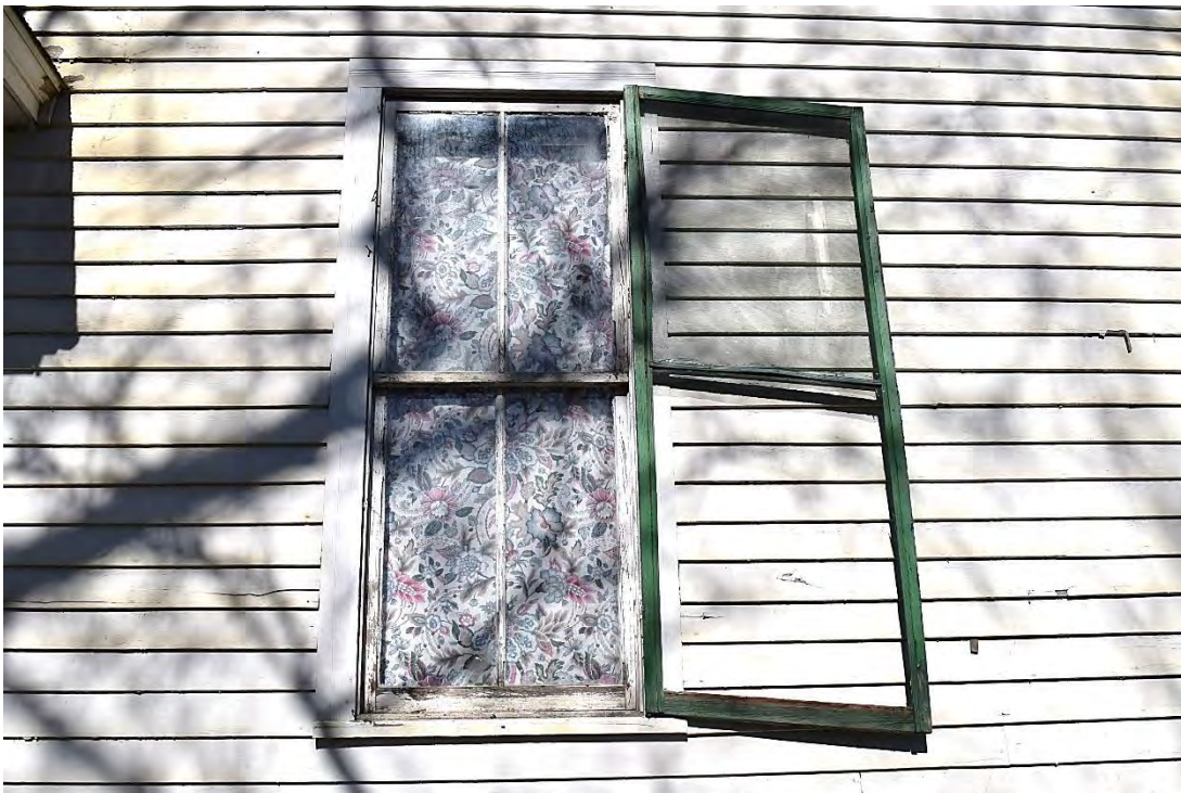
McLaughlin-Bost House, Side (East) Elevation, Window, Looking West.
