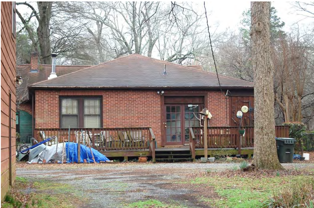
John and Roselie Stewart House, Rear (North) Elevation, Looking Southwest.
