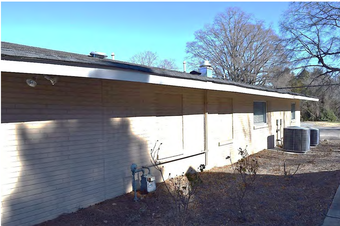
Medical Office Building, Side (South) Elevation, Looking North.
