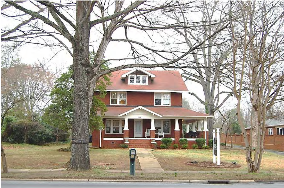
Renfrow-Lemmond House, Overall View, Looking North From West John Street.
