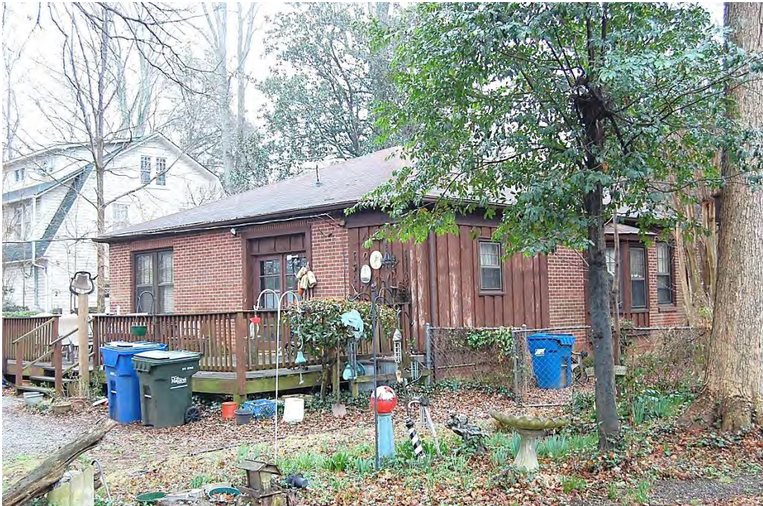
John and Roselie Stewart House, Rear (North) and Side (West) Elevations, Looking South.
