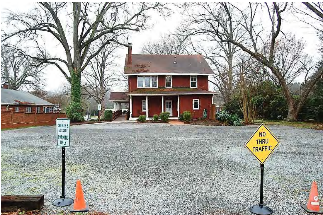
Renfrow-Lemmond House, Rear (North) Elevation and Parking Lot, Looking South.
