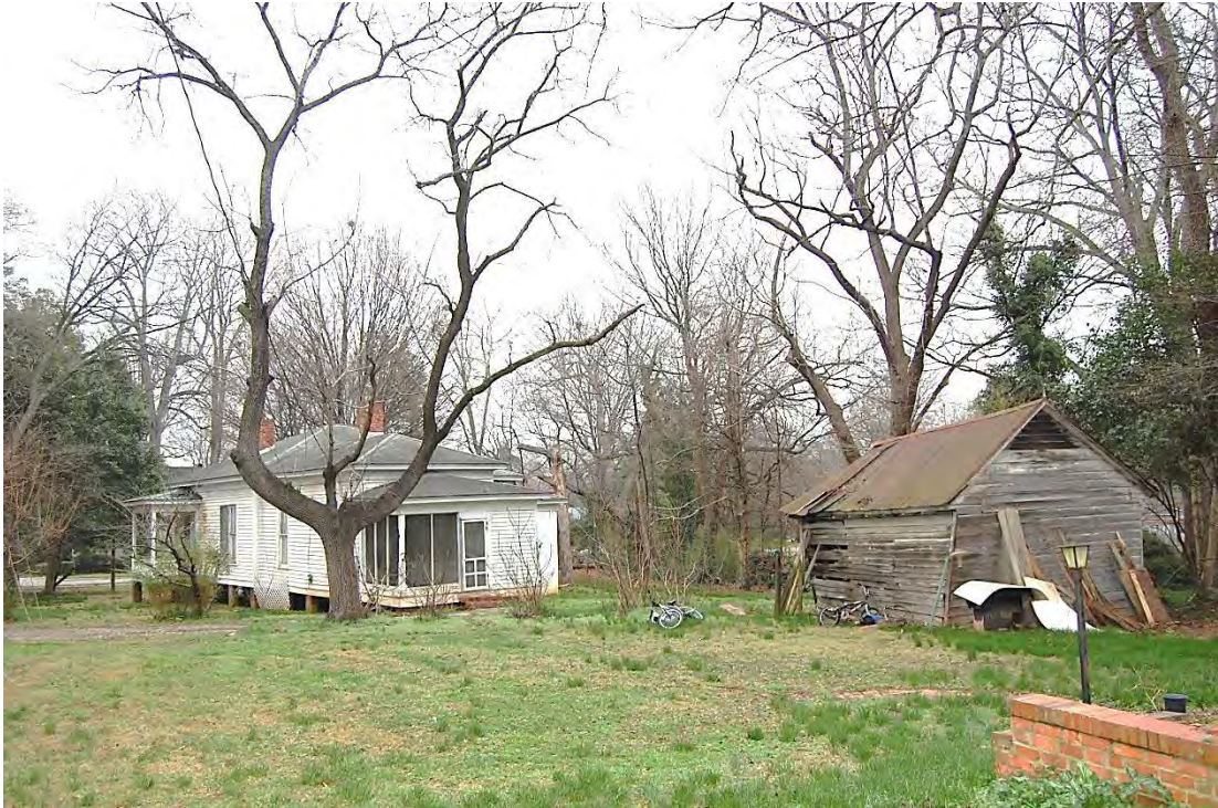
McLaughlin-Bost House, House and Deteriorated Garage, Looking Northeast.
