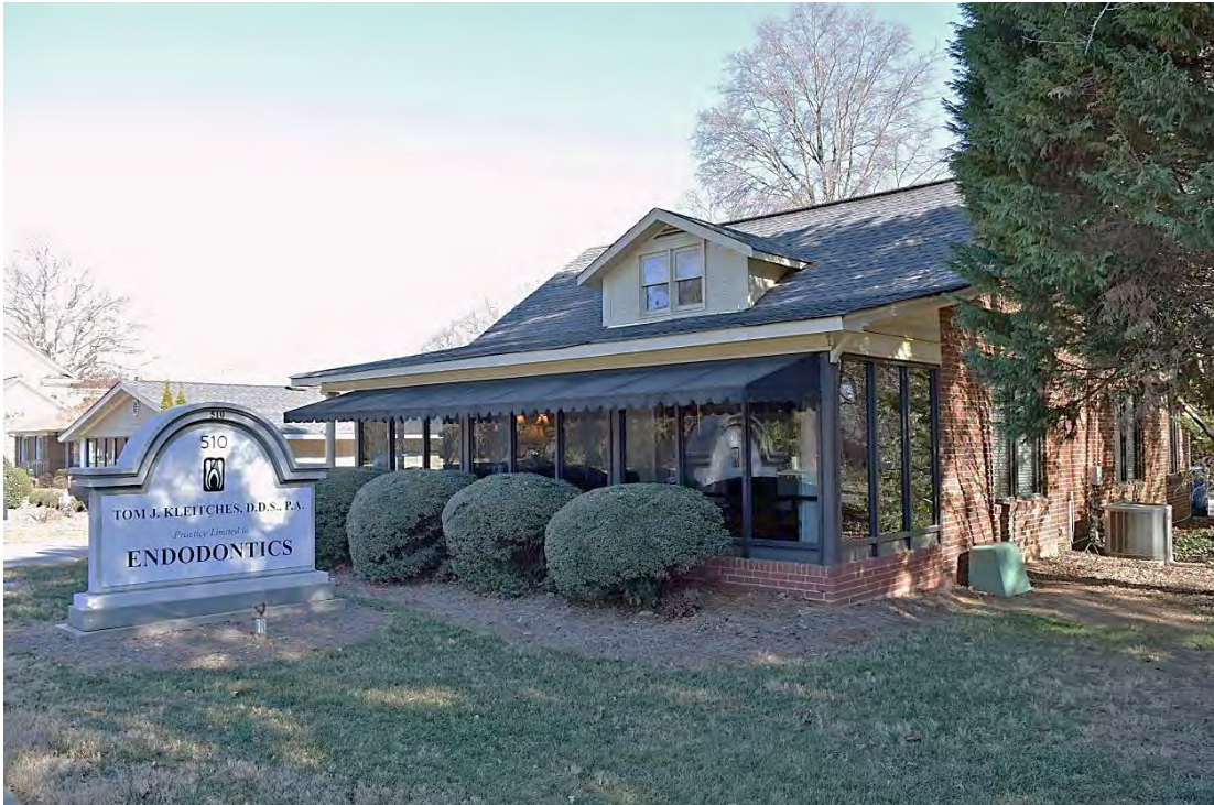
Jesse and Ethel Hartis House, Façade, Looking North.
