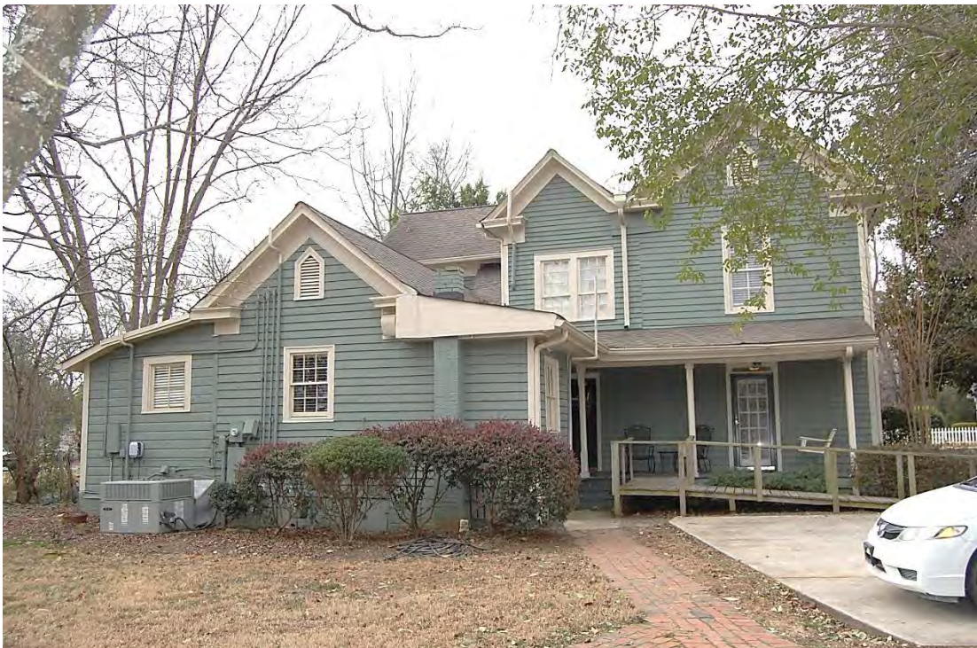
Grier-Furr House, Rear (East) Elevation, Looking West.
