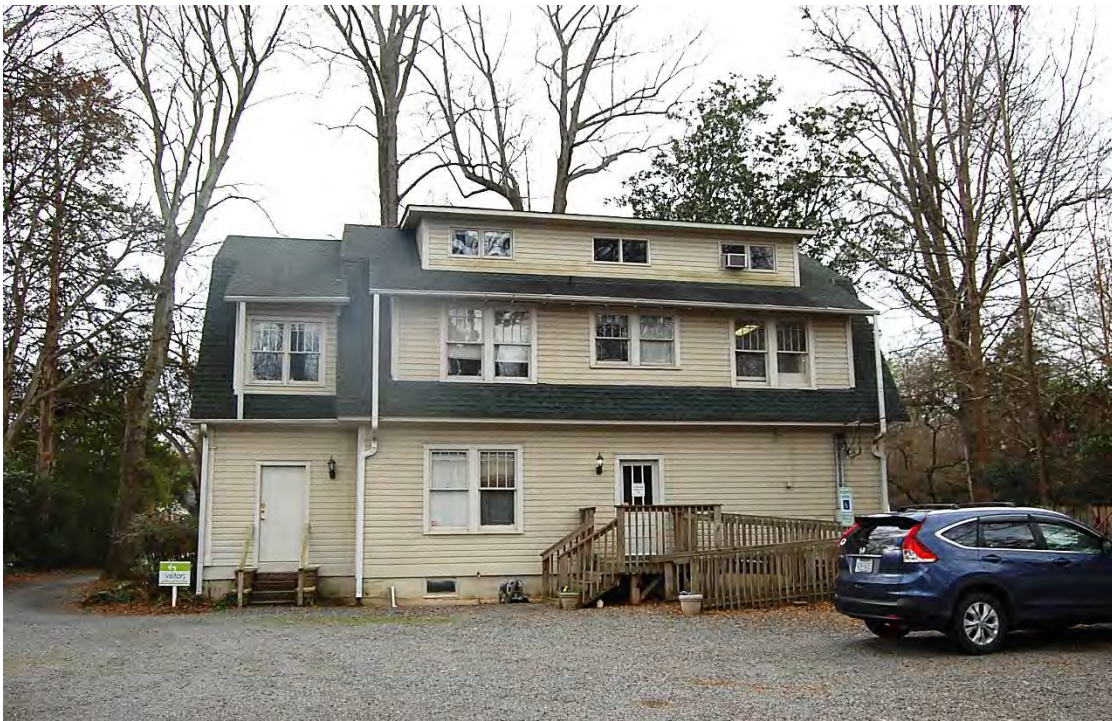
Kidd-Tennant-Roberts House, Rear (North) Elevation, Looking South.
